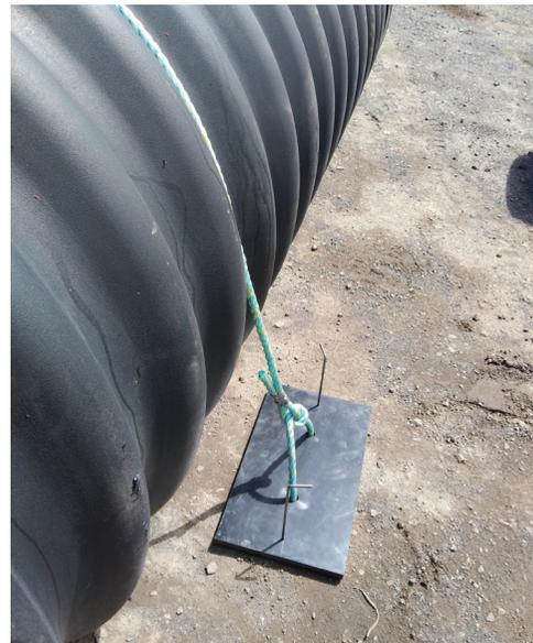
New slimmer design 300mm wide anchors for narrower trenches. Securing pegs now provided to secure pads in place to prevent pad slippage when backfilling!
